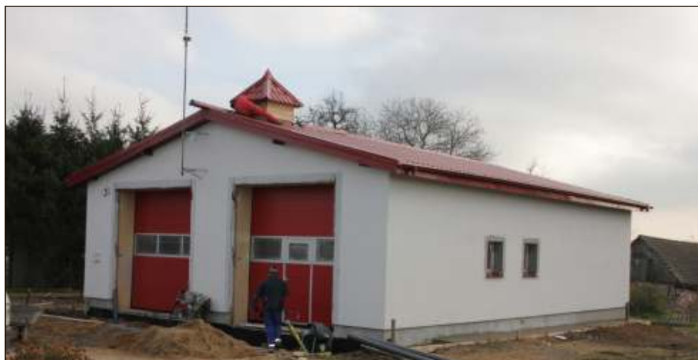
Remont remizy OSP Karsino
